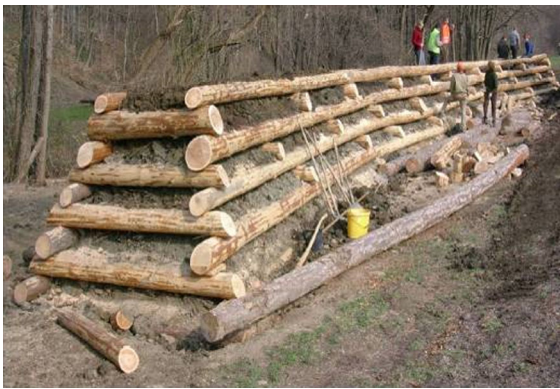
Fig. 2 Wooden log crib wall for noise control in Lower Austria (March 2004)
