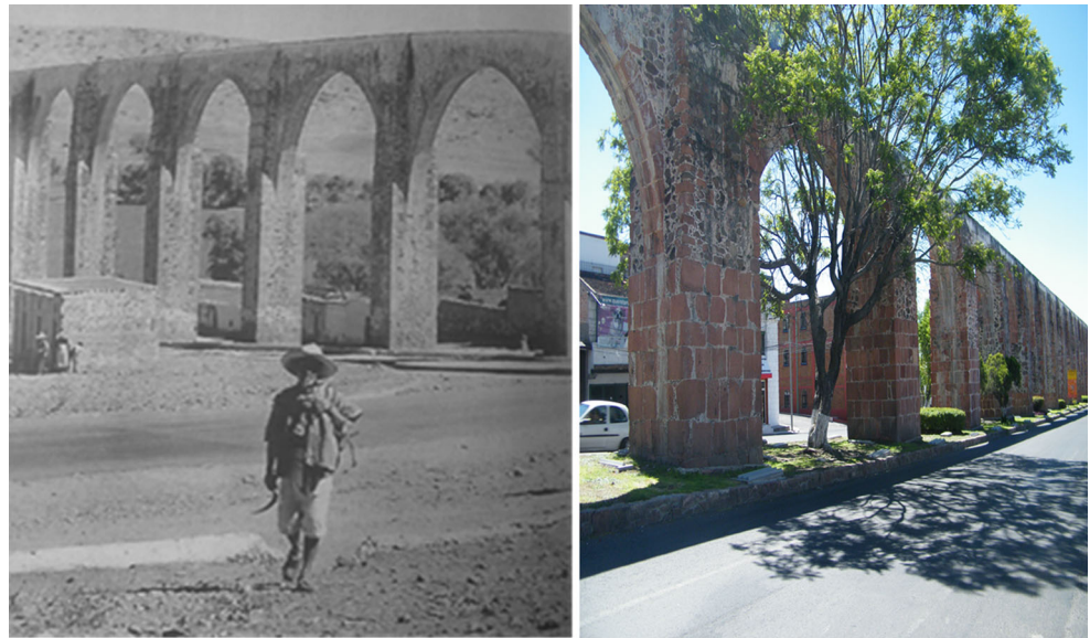
Fig. 1 The Arches , the most representative part of the aqueduct in Queretaro, Mexico. At the beginning of the twentieth century ( left ) [5], and their current status ( right )
