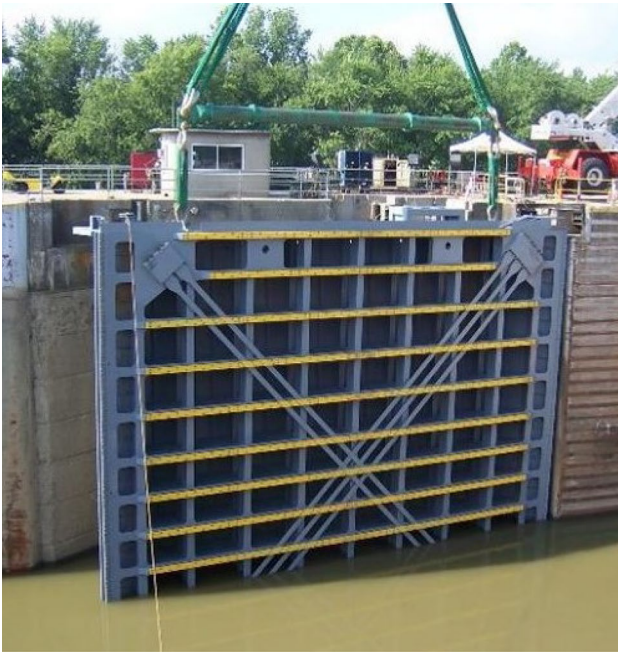
Fig. 1 An open miter gate
