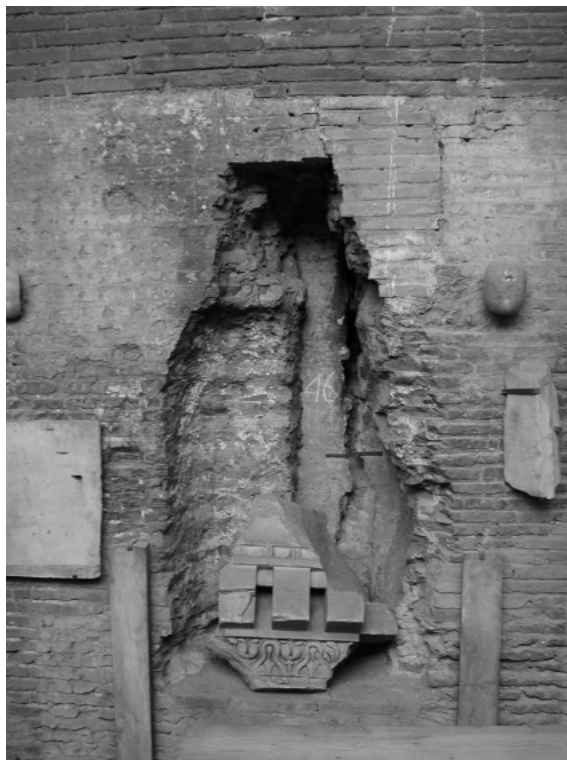
Fig. 3. Pantheon, upper floor, view to the east. The photograph shows the room of the nave which probably housed the Bibliotheca Alexandrina in the third century. The Rotunda lies behind the brickwork filling the side arch to the north. The upper string course of the cornice of the Rotunda is at the height of this floor. This is where the dome springs, and in which, in the lower bricked-up opening at a depth of roughly two feet, an area of one-half square meter has been opened. building inspectors found a crack here in the cement covering which was caused by shrinkage during the construction of the dome. Above this point there is another vertical opening in the brickwork roughly 3 m. long and 1/2 m. deep. It was later bricked up in a way that is clearly different from the original construction. An opening to the dome might have been here. As the wall slit is placed very near to the south of the Rotunda, it would be perfectly positioned as an observation point to the north for measuring the circumpolar sky above the oculus. This observation post lying next to the room that is believed to have housed the Bibliotheca Alexandrina, supports the hypothesis that the study of the universe was, from the very beginning, part of every important book collection.
