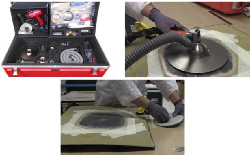
Fig. 5.10 Illustration of the stepping process prior to the application of a repair patch in the bonded repair user case
