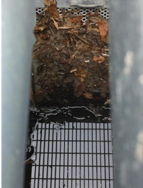
**Fig. 6.11** This picture shows mesh screen in an underground detention tank fully blocked, preventing design discharge
