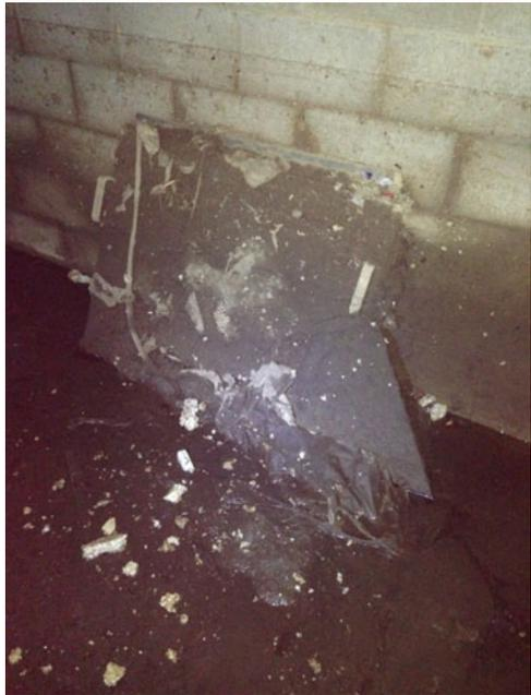
**Fig. 6.12** This picture shows a mesh screen, which is unsecured to the walls of an underground detention tank with some of the trash collected whilst smaller materials were allowed to be released
