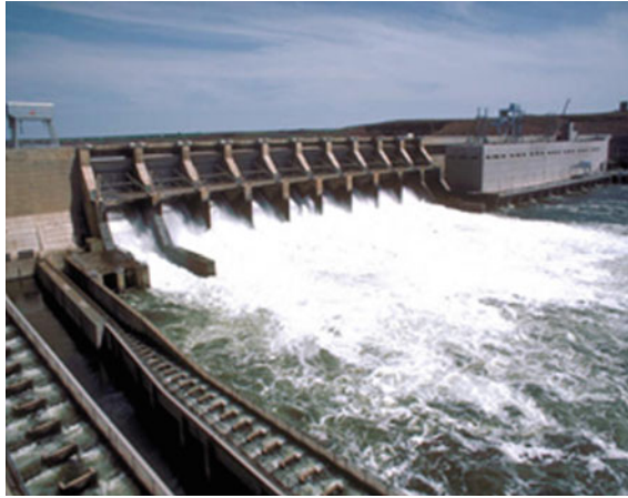
Fig. 2.5 Ice Harbor Dam. Hydroelectric plants operate where suitable waterways are available. Water may be a source of cheap and relatively clean power. In addition, because there is no fuel combustion, there is little air pollution in comparison with fossil fuel plants and limited thermal pollution compared with nuclear plants. The use of water for power generation has environmental impacts caused by damming rivers and streams, which affects the habitats of the local plant, fish, and animal life [14]
