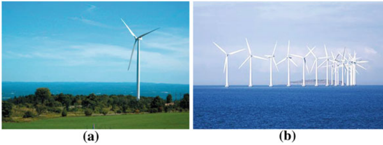
Fig. 2.14 a Each 1.65 MW wind turbine at the Maple Ridge Wind Farm near Lowville, New York, generates enough electricity to power about 500 homes. Jennifer Harvey, NYSERDA, NREL PIX 14399; b offshore wind resources. Currently, the US has more than 35,000 MW of land-based installed wind power capacity. That is enough to serve more than 9 million homes and avoid the annual emissions of 62 million tons of carbon dioxide [13]
