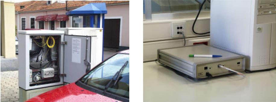
**Fig. 6.** BBL AS-ONU mounted on a street cabinet and a VDSL modem (NT-51).
