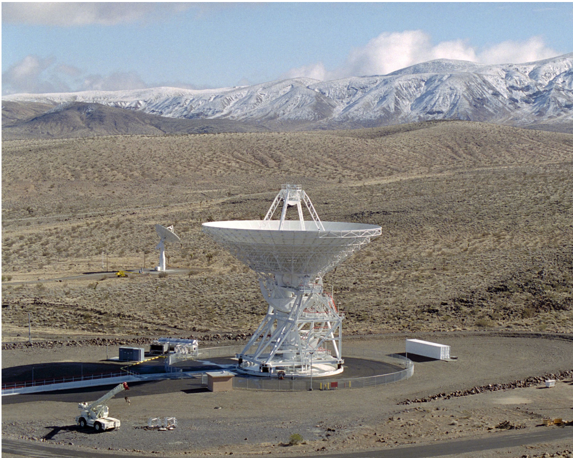
Figure 3: DSS 25, a 34-m beam-waveguide antenna, shown here in the stowed position. DSS 25 is one antenna in the NASA/JPL Goldstone Deep Space Communications Complex near Barstow, CA, U.S.A. It has special instrumentation (Ka-band up- and downlink and advanced tropospheric calibration capability) which enable particularly good quality Doppler observations.
