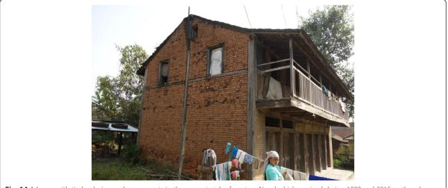
Fig. 14 A house with timber lacing and corner posts in the same stretch of western Nepal which survived during 1988 and 2015 earthquakes
