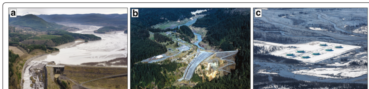
Figure 8 Examples of large-scale lahar containment and exclusion structures. (a) The Sediment Retention Structure (SRS) downstream of Mount St. Helens, USA, built specifically to contain potential lahars and eroded sediment (USGS photo by Adam Mosbrucker, 11 Nov 2012); the volcano is visible on the horizon on the left side of the image. (b) Mud Mountain Dam with a large concrete overflow spillway on the White River downstream of Mount Rainier (USA), (Stein 2001). It was built as a flood-control structure but it also may function as a trap for at least part of future lahars because little water is normally impounded behind the dam (photo courtesy of U.S. Army Corps of Engineers). (c) Exclusion levees surrounding the Drift River oil terminal on an alluvial plain approximately 40 km downstream of Redoubt Volcano, Alaska (USGS photo by Chris Waythomas, 4 Apr 2009).
