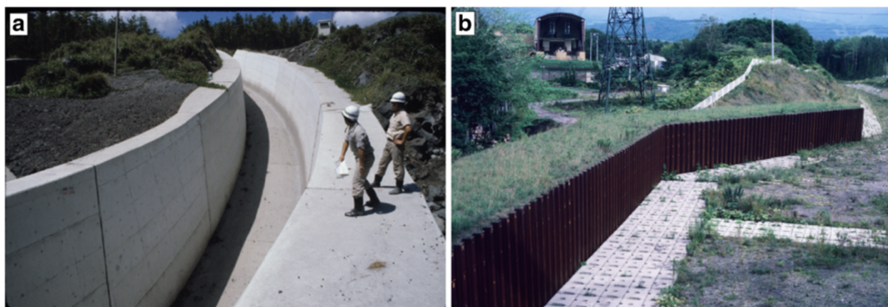
Figure 7 Types of lahar diversion structures. (A) Engineered channel reach in small river draining Sakurajima volcano in southern Japan, where channel is revetted with reinforced concrete and engineered to be as steep, narrow, and smooth as possible, in order to divert lahars away from a developed area. (B) Training dike revetted with steel sheet piles on the lower flank of Usu volcano, Japan and designed to deflect lahars away from buildings and other infrastructure. USGS photos by TCP.
