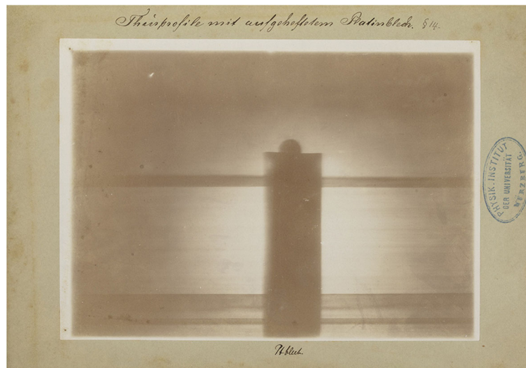
Fig. 4 The doorpost of Roentgen's lab upon which he attached a thin sheet of Platinum. It shows that the X-ray attenuation of the thin plate of platinum is much larger than that of the thick wooden doorpost. Manually written legend: 'Thürprofile mit aufgeheftetem Platinblech' (Doorpost with attached thin plate of Platinum). Paragraph referral: § 14
