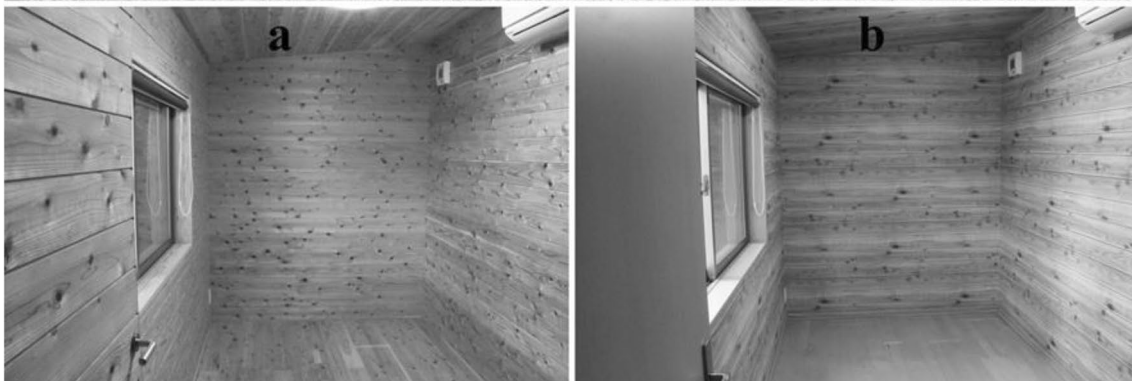
Fig. 1 The layout of the experimental houses and photos of (a) Room A, and (b) Room B at Kyushu University. The interior of Room A was composed of planed Japanese cedar lumber, and Room B had printed grain resin sheet overlay boards
