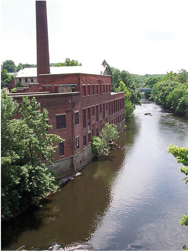
Figure 6 Former textile mill along the Blackstone River in the Blackstone River Valley National Heritage Corridor (Source: U.S. National Park Service).
