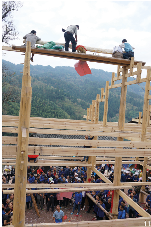
Figure 10 'The precious beam' is under a ridge beam. Zaidang Village, 2017 (Source: Congcong Ren).
