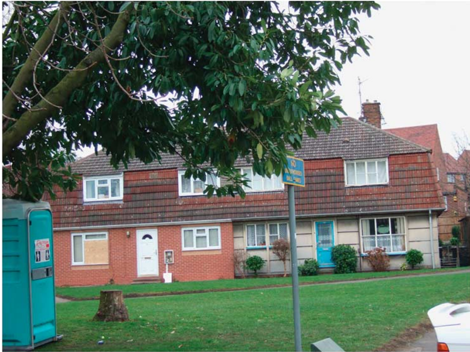
Figure 1: Original construction of small pre-cast concrete panels supported by pre-cast columns (right) and overladded with brick (left).
