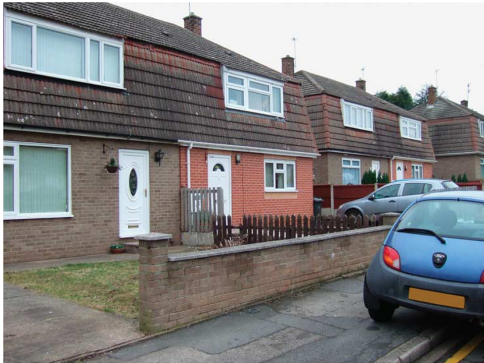
Figure 2: Once face-lifted with brick cladding and new UPVC fenestration, they can be made aesthetically attractive.
