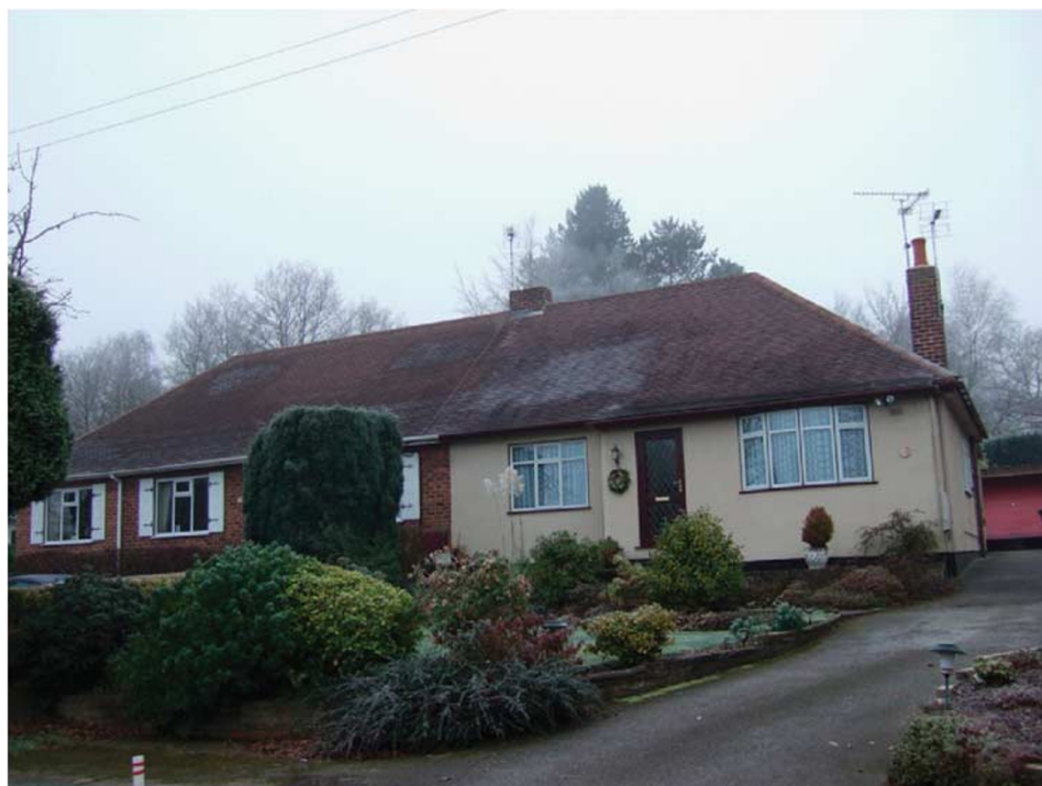
Figure 4: A pair of originally prefabricated semi-detached properties dating from the late 1950s which have evolved differently.
