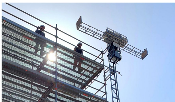
Fig. 5 Kewazo's Liftbot scaffolding assembly robot
