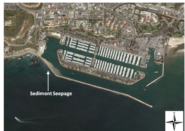
Fig. 11 Google Earth photograph of Dana Point Harbor taken in April 2005
