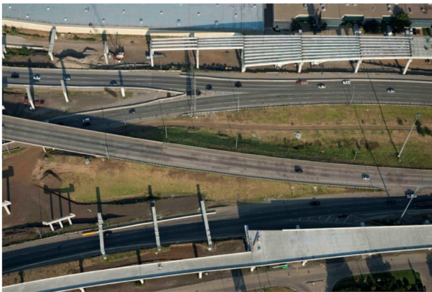
Fig. 4 Bridge 4 construction, bent caps 7, 8 and 9 in place
