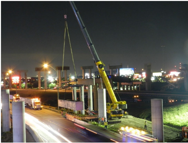
Fig. 15 Lifting of composite bent cap
