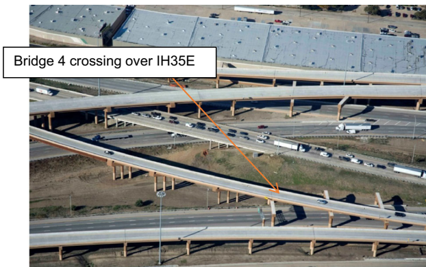
Fig. 2 Bridge 4 crossing over IH-35E, in service
