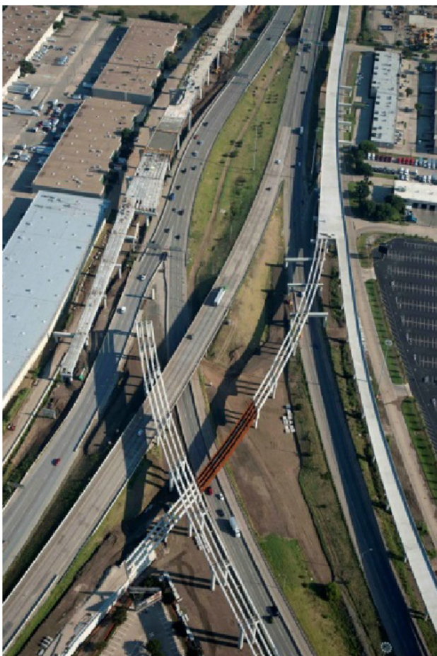
Fig. 5 Bridge 4 construction, girders in place
