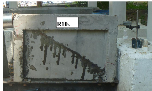
Fig. 10 Epoxy repaired, with concrete infill diagonal braced frame
