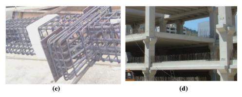
Fig. 1 A precast structure under construction with hybrid beam-column connections. a Welding of longitudinal beam bottom rebars to beam end plate. b Installation of flexural and shear reinforcement for a precast beam. c Installation of flexural and shear reinforcements to constitute the precast column and corbels. d Assembling precast beam and column elements on site.
