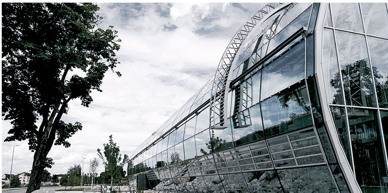
The global R&D center in Trostberg (Germany) is the heart of the innovation chain for admixture systems, underground construction, and resins.
