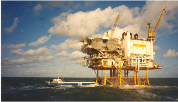
Fig. 1 Photo of the MS Reint-H7 allision, taken by the crew on the nearby standby vessel
