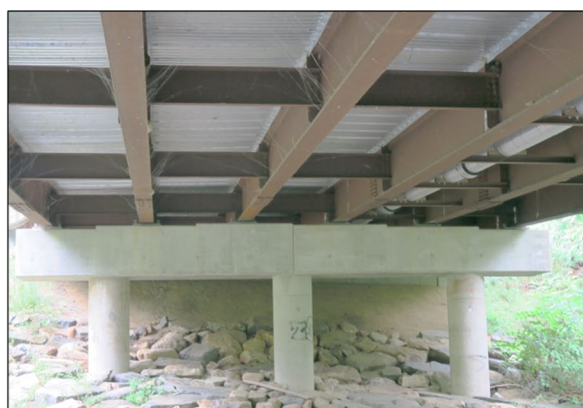
b) Underside of the bridge
