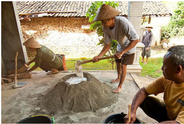
Fig. 2 Mixing of the mortar in-situ
