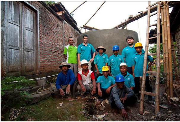
Fig. 12 Group picture after finishing of the cistern construction using the developed material concept
