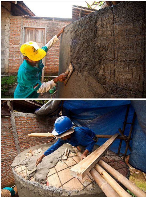
Fig. 4 Application of the outer mortar layer ( top ) and application of the mortar on the ceiling ( bottom )
