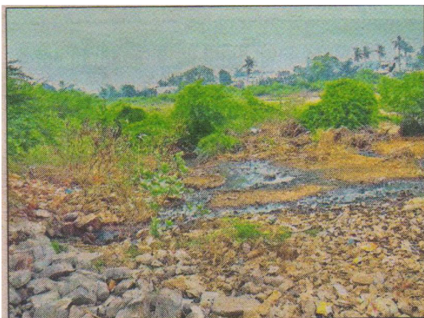
Fig. 23 Drainage fed into Champavathi River
