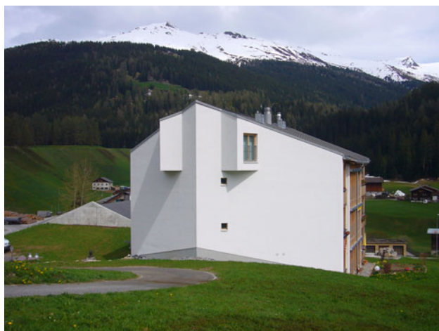
Fig. 10 Splitting wedge directly connected to the exposed object (Davos Frauenkirch, Switzerland)
