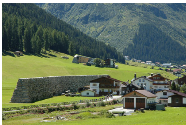
Fig. 11 A deflection wall used to protect an entire building ensemble from the impact of medium-magnitude events (Galtür Tschafain, Austria)
