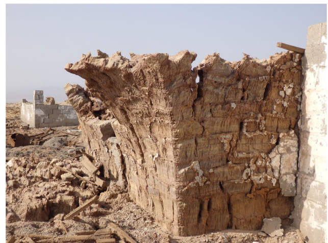
Fig. 5 Remains of the Parsons Mining Camp made from blocks of layered Dallol salt, now slowly falling apart and inclining. Note the straight concrete block building in the background as a contrast
