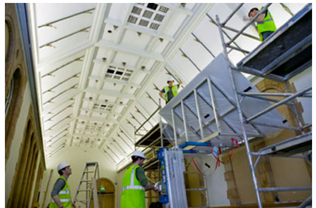
The newly refurbished gallery with ceiling armatures for the 18 panels in place: receiving the first panel
