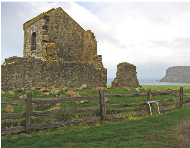
Fig. 5 The ruins of the convict barracks at Highfield in the far North West of the state were part of the Van Diemen’s Land Company holdings
