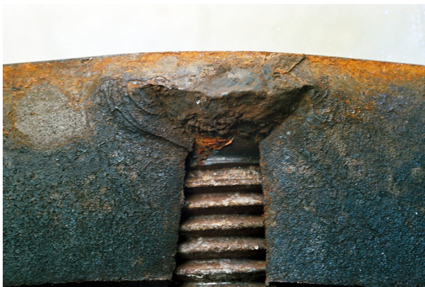
Fig. 14 Crack shown in Fig. 13 now opened to expose screw as-installed and related fatigue crack surface
