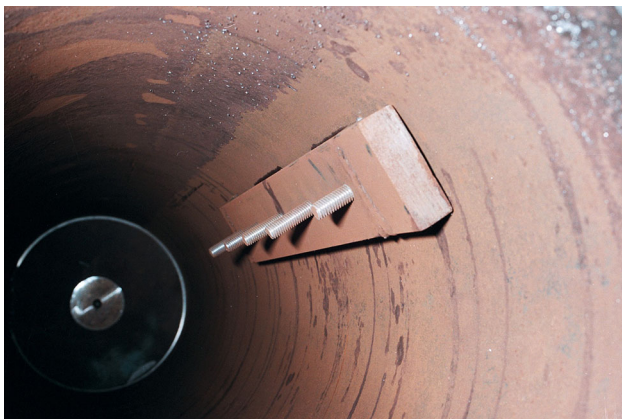
Fig. 5 Another balance weight installed on long end of fractured roll
