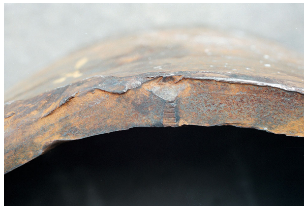
Fig. 7 Close-up of fracture origin (see Arrow 1, Fig. 4)
