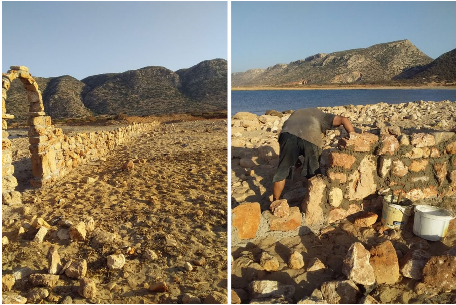
Fig. 10 Perimeter wall constructed around Sidi Awlad Noah to mark the outline of the site to protect it from future development
