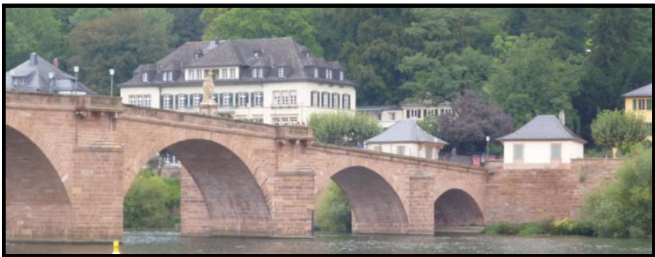
Fig. 2 The bridge across the Neckar River connecting the town with the residential hillside, as discussed by Heidegger (1950/1967). Photo: G. Stahl, Heidelberg, Germany, 2012
