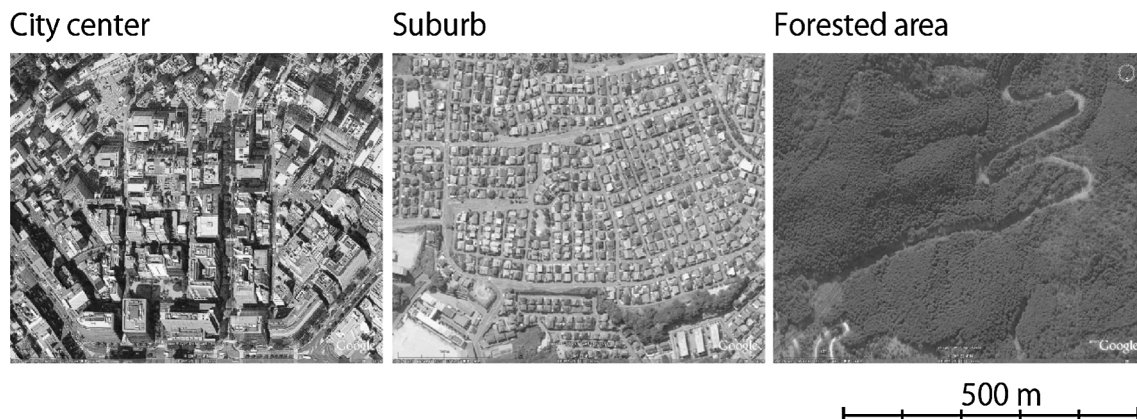
Fig. 2 Aerial photographs illustrating the features of the three studied environments (from Google Earth)
