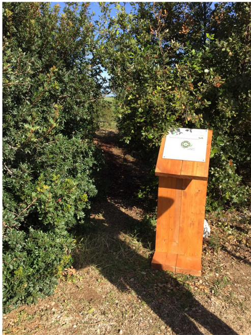
Fig. 9 The wooden installations a wooden structure consisting of an element (2.15 * 0.08 m), including hardware and poles to be driven into the ground for a minimum depth and suitably anchored to the panel to avoid creating the sail effect due to the action of the wind and any other horizontal component acting on the panel. To this end, the pile is founded with a system of wooden foundations, fine and coarse gravel, sand. Forex panels (5 slabs of 0.1*0.40*0.02 m) have been applied to the supporting structure, hooked to the structure, which direct the visitor towards the “green rooms” designed for Villa Framarino. A tactile map with Braille translation completes the georeferencing information indicating the exact point where you are with respect to Villa Framarino building and the green rooms with respect to this entry point
