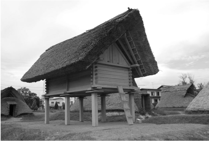
Fig. 3 A reconstructed example of a Yayoi ‘raised-floor rice granary’ at the Toro site (reproduced with permission of Shizuoka City Museum, Shizuoka Prefecture, Japan)
