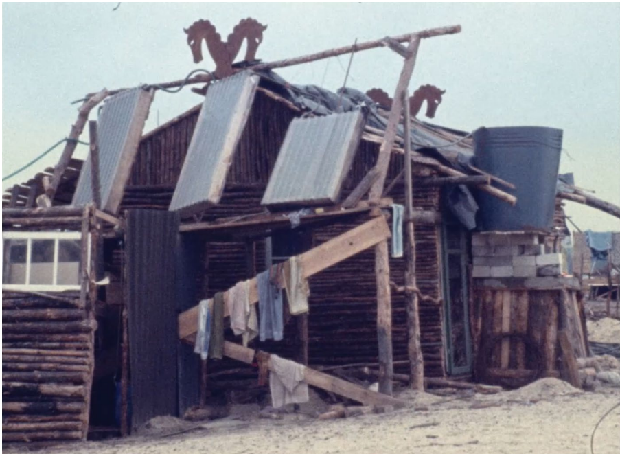
Fig. 4 Early experiments with solar energy providing warm water for the collective bathroom, May 1980 (Wendländische Filmkooperative 1981:83mins36sec)
