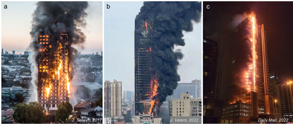
Figure 1. Typical facade fires in the high-rise building, (a) Grenfell Tower fire, London, UK, 2017, (b) Communication Tower fire, Changsha, China, 2022, and (c) Boulevard Walk Tower fire, Dubai, UAE, 2022.
