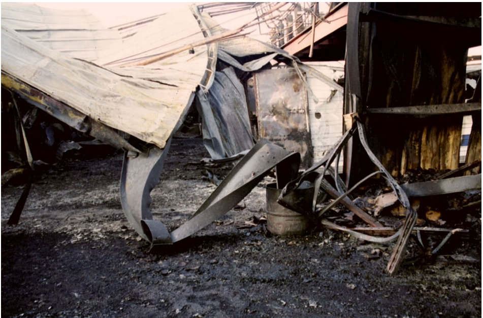
Figure 3. Column A7 adjacent to the loading bay.
