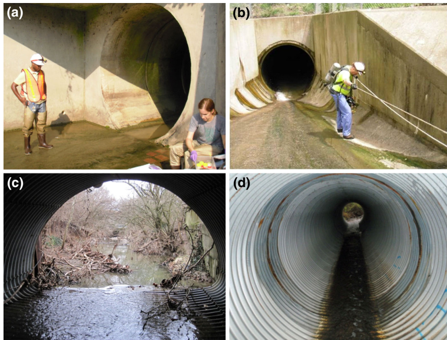
Fig. 2 Pictures of buried streams included in this study. Este (EST) (a, b) flowed through a concrete tunnel with a narrow wetted width at baseflow. Amberly (AMB) (c) flowed through a wide corrugated metal pipe which was filled with sediment to a
