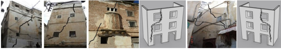
Fig. 11 In plane mechanism
