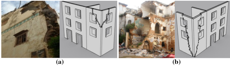
Fig. 9 Overturning a partial combined mechanism, b total combined mechanism
