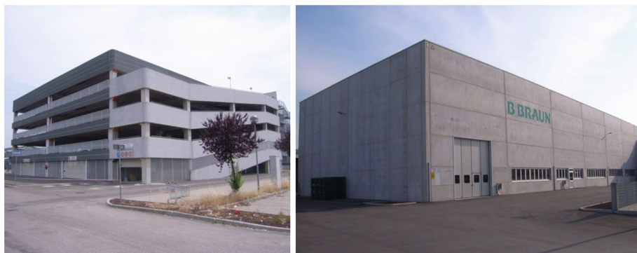
Fig. 13 Recently constructed precast concrete buildings exhibiting good performance
