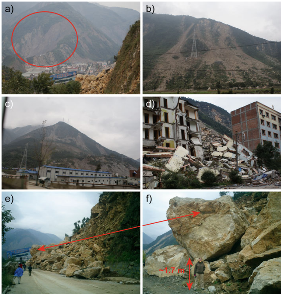
Fig. 17 Landslides and rock falls in Beichuan. a–c Landslide scarps visible on the steep mountain slopes surrounding Beichuan. Temporary shelters are visible in the foreground of (c) . d Landslide in the center of Beichuan, causing an apartment block to total collapse. To the right a building with no apparent damage is visible. e–f Large rock falls and boulders blocking the road to Beichuan, notice the huge size of the boulder in (f)
