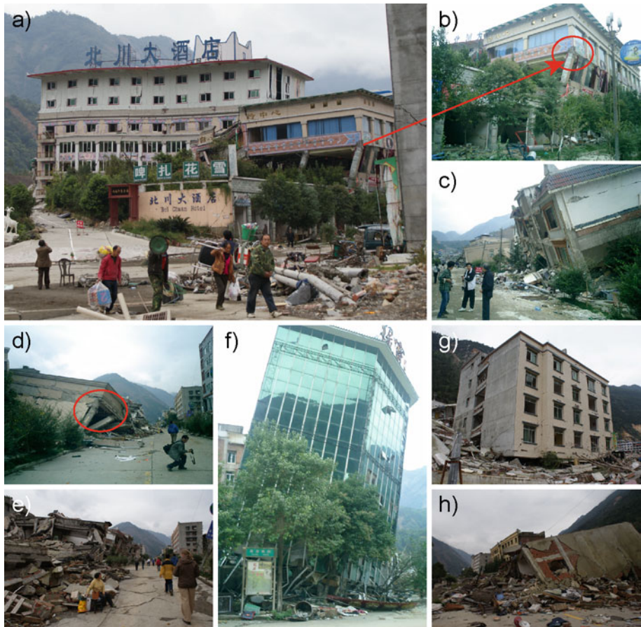
Fig. 10 Building damage in Beichuan County Town. a–b Bei Chuan Hotel suffered severe damage, as failure of the column beam joints, but sustained the ground shaking. The main building of the hotel is clearly tilted ( a ). c–e Main street of the newer part of Beichuan, with collapse of weak structures due to column failure. f–g Buildings suffering single story collapse of the first floor. h Toppled building due to ground failure
