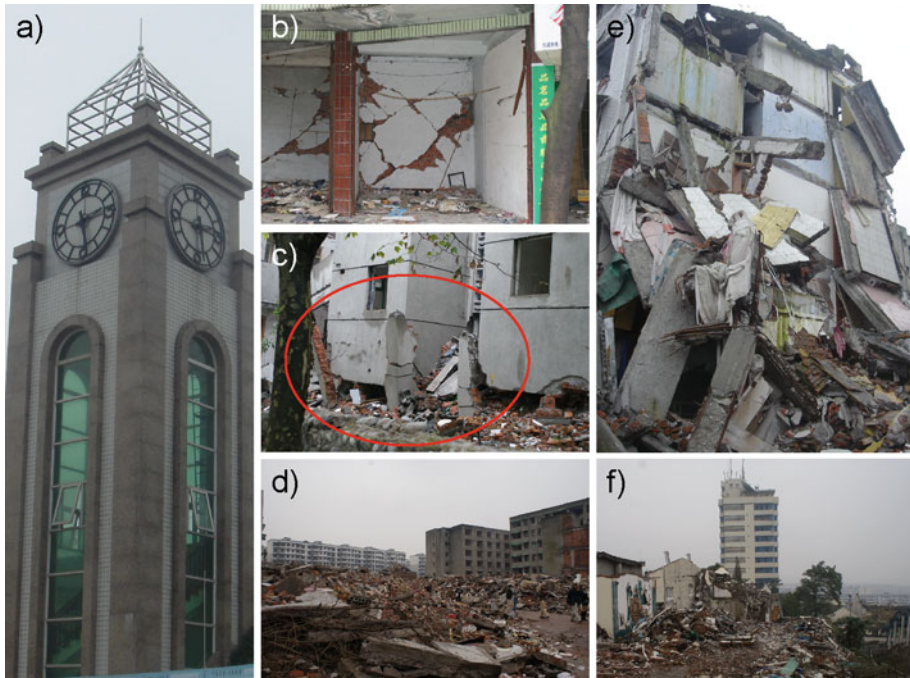
Fig. 7 Building damage in Hanwang. a City clock tower of Hanwang with no apparent damage. The clock stopped at the time of the earthquake, 14.28 (local time). b View inside a building, with visible non-structural damage. c Single story collapse of apartment building. d–e Widespread damage of poorly constructed buildings, whereas modern buildings sustained the ground shaking. f Main building of Dong Fang Steam Factory with no apparent damage. In the foreground widespread damage and collapse of poorly constructed buildings is visible
