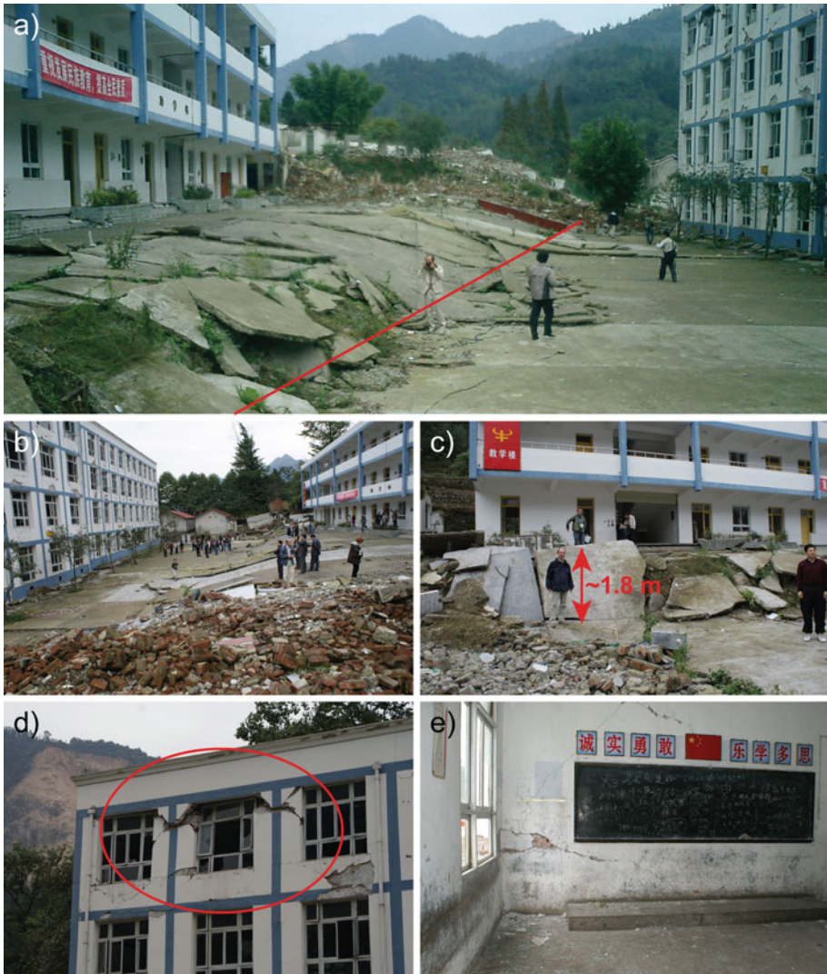
Fig. 5 Damage of Bailu Middle School buildings and fault scarp in Bailu. a–b School yard, taken towards northeast and southwest, respectively. c Newer school building on the hanging wall block with no visible damage. Vertical uplift of approximately 1.8 m is visible. d Structural failure of cross diagonal fractures on the older school building. e View from inside the older school building, where wall cracks are visible
