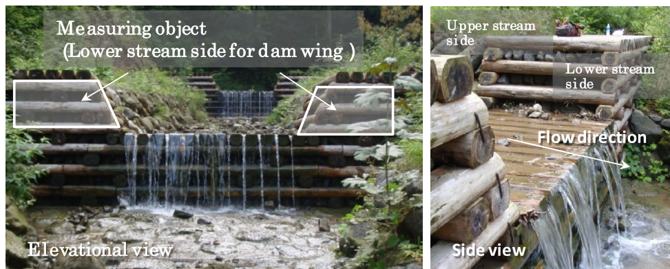
Fig. 2 Positions of the components for which decay was measured (Shusuicho Dam, Fujinomiya City, Shizuoka Prefecture)
