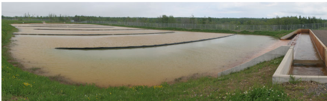
Fig. 3 View of the settling pond with the five baffle sheets installed (2010-06-21)
