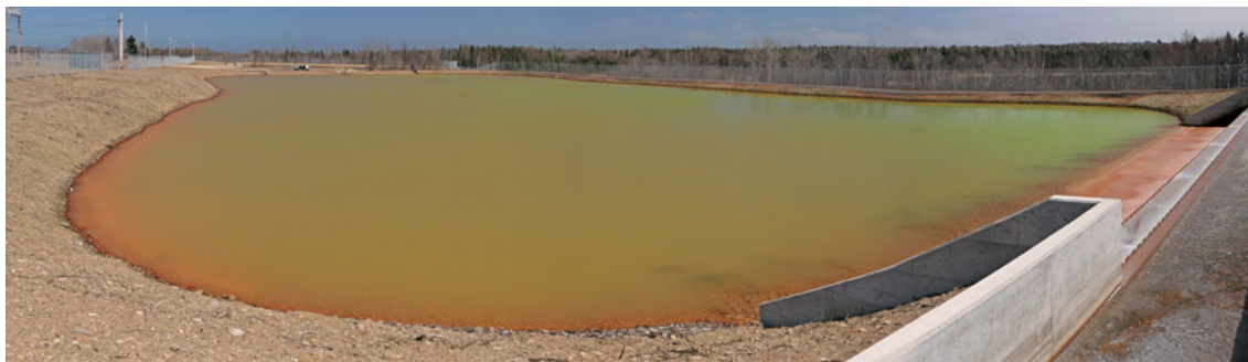
Fig. 2 View of the Neville Street settling pond with the mine water inflow (CPI) and cascade on the right and the outflow (OSP) in the upper left corner . Length of the settling pond 150 m, width 60 m (2009-05-12, before the installation of the baffle sheets)
