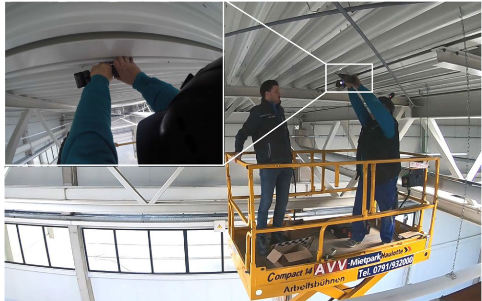
Fig. 6 Installation of cable clamps recorded in the long shot and from the users view (left corner)
