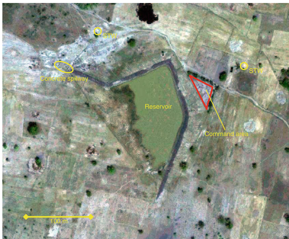
Fig. 2 Satellite image of the micro-dam irrigation scheme
