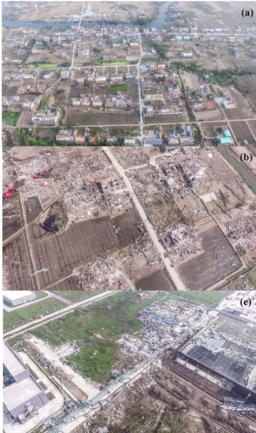
Fig. 1. Aerial survey images showing extensive and severe damage caused by the Funing County, Yancheng City, Jiangsu Province tornado of 23 July 2016.
