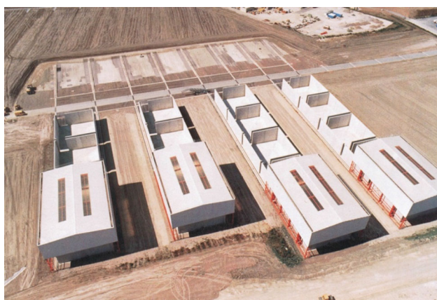
Fig. 2 Photograph of the Centre de l'Aube (France) surface repository for LLW (low-level waste). Waste packages will be placed in the large, open concrete compartments (mid-field) and, after they are full, each will be closed with a concrete roof and the entire site then covered with an earth and clay 'cap'. Image courtesy of Nagra
