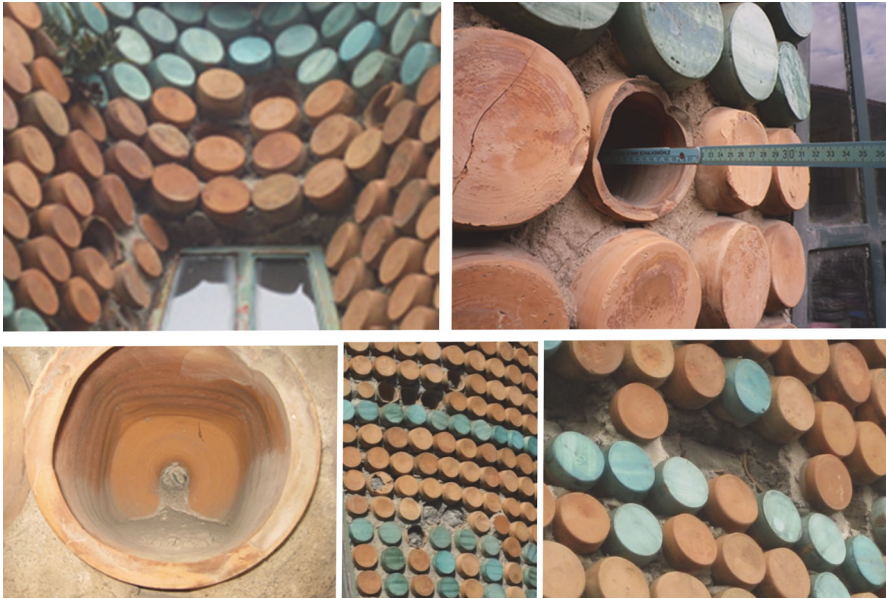
Fig. 4 Details of the exterior facing on the south façade. Photos: author
